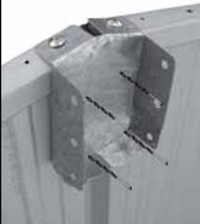
Looking from inside of the shed
