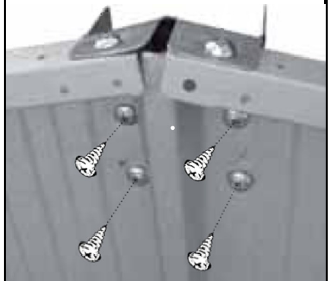
Looking from outside of the shed
